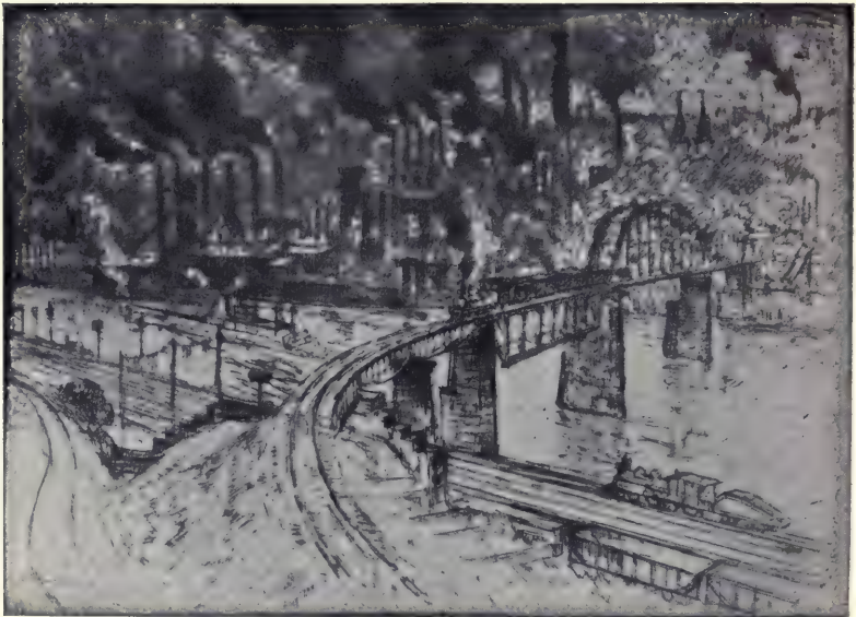
THE CURVING BRIDGE, PITTSBURGH Size of the original print, 8 by 11 inches. From the etchings by Joseph Pennell.
